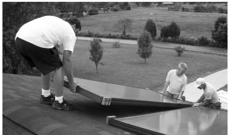
Jeremy Coxon (center) instructs HFH crew on solar water heater installation
